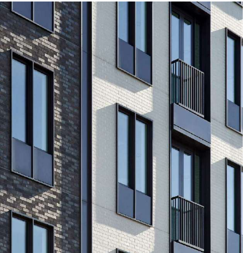
Farrells pre cast masonry panels with texture and variety at Royal Albert Docks
