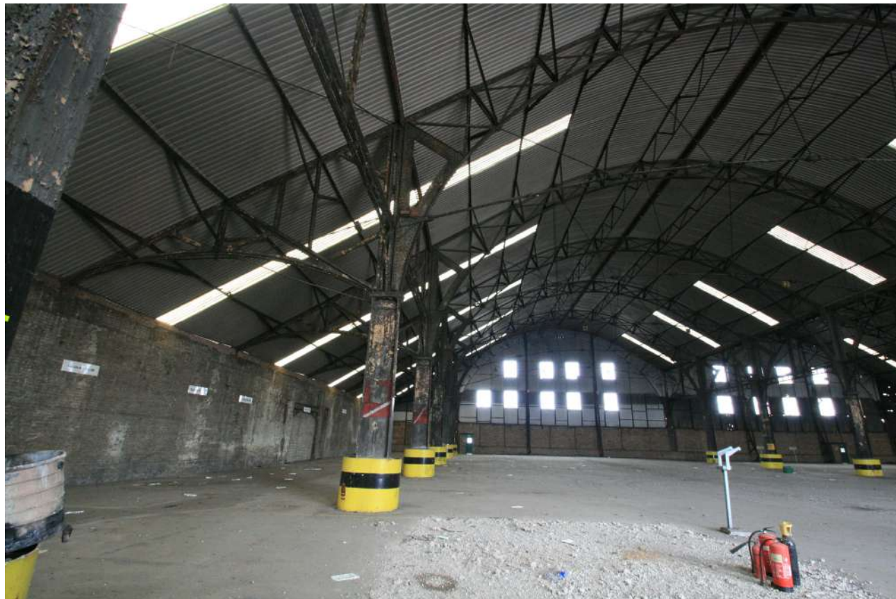
Olympia Building - Industrial Metal Structural Frame
