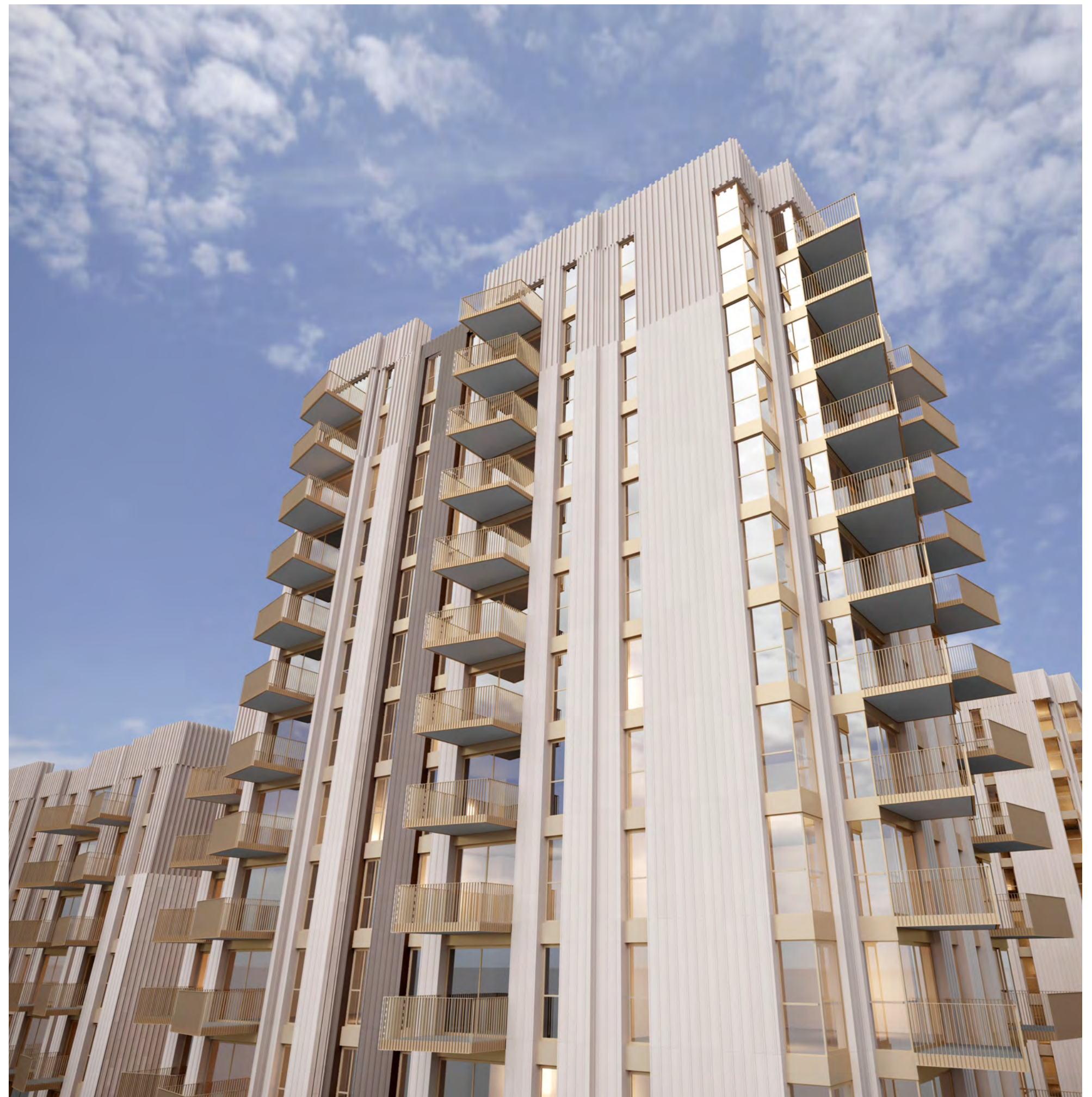
Change in panel grain and relief of panels at upper level to visually define the building top. Facade recesses visually emphasised with change of terracotta tone, panel size and reduced parapet height.
